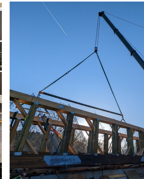
ENR BEST OF THE BEST SMALL PROJECT CATEGORY Spellacy Bridge Reconstruction
